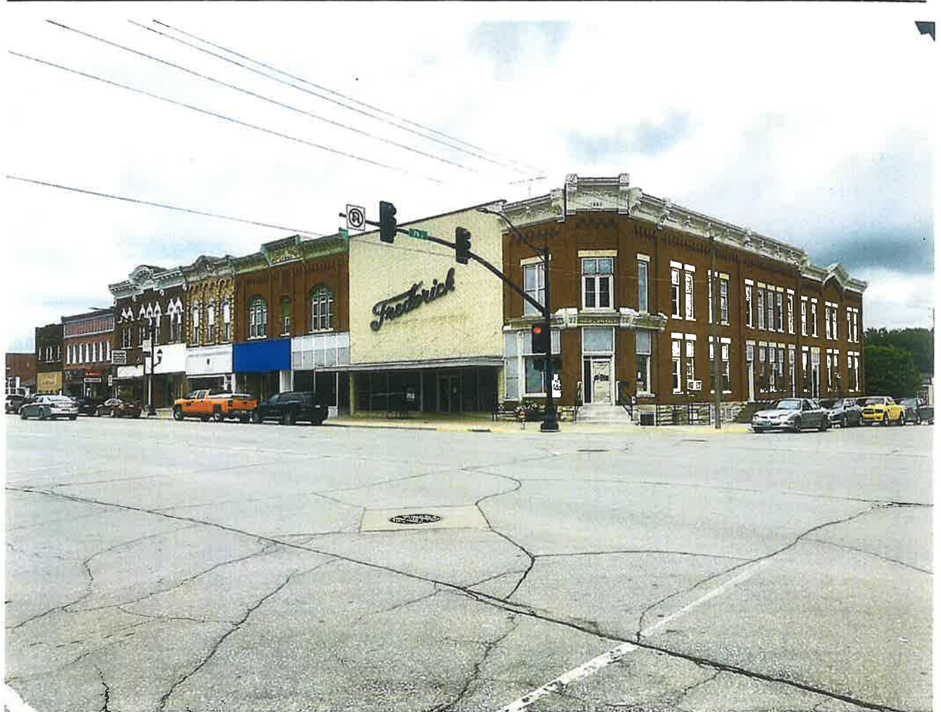
General view northwest
