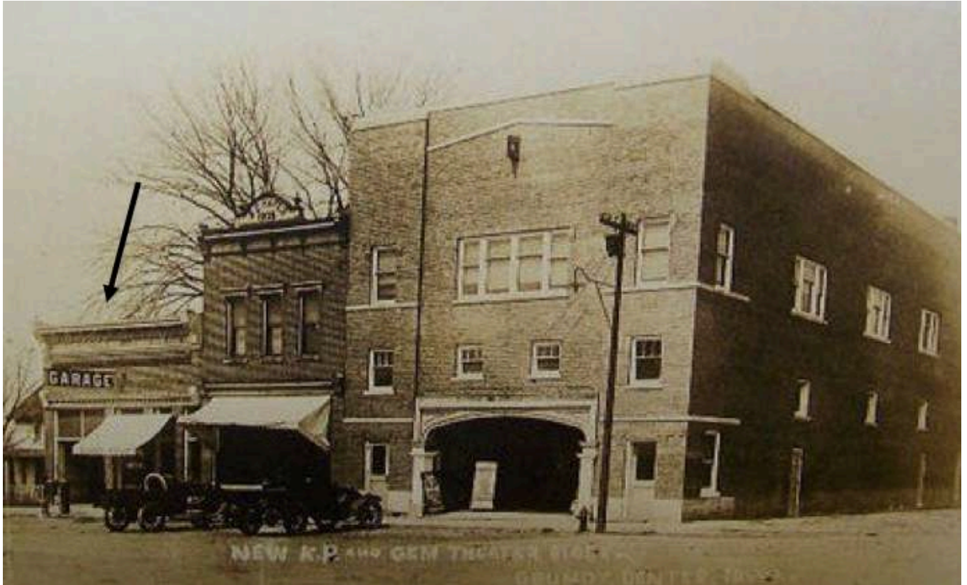
View northwest of Schafer Garage (arrow) next to nonextant Gem Theater, 1912 Source: Grundy County IAGenWeb
