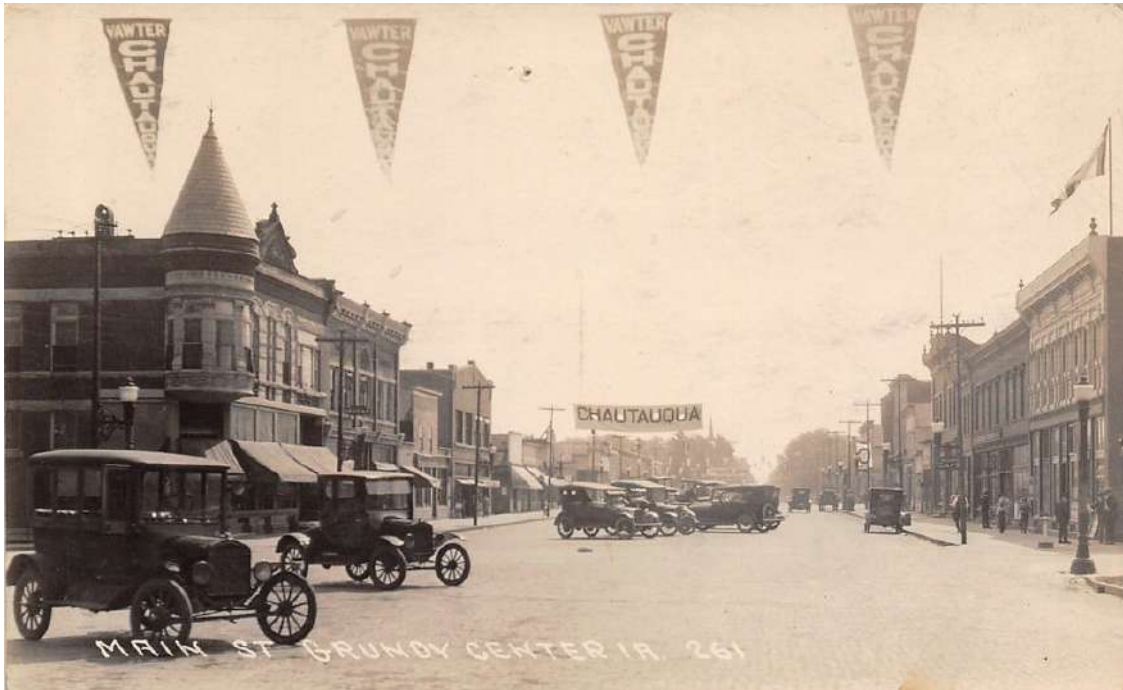
View northeast, c.1915, with Hummel Block on left Source: Grundy County IAGenWeb
